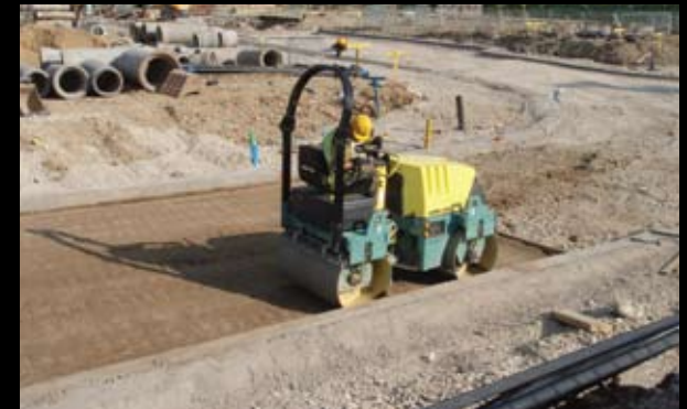
Compaction of PVX-6® replacing bituminous material to form the road base.
