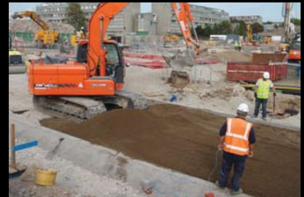
Spreading and levelling of PVI® replacing Type 1 to form the sub-base.
